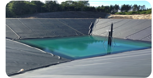
Sensible TES with water in pit
