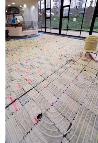
Floor heating with PCM Cesari et al., 2024
