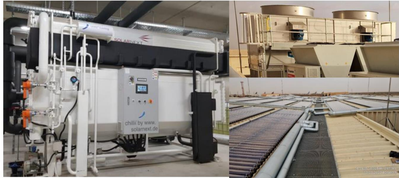
Figure 2: Lithium bromide absorption chiller with closed circuit cooler and vacuum tube solar collector field (from left to right), Sources: SolarNext.
